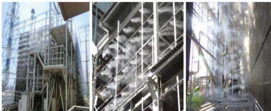
Figure 4: Fogging inlet cooling systems
