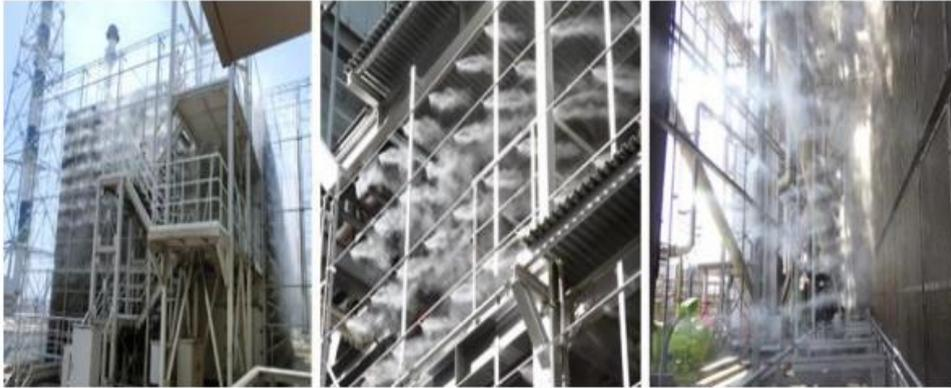
Figure 4: Fogging inlet cooling systems
